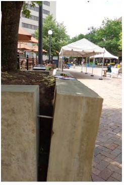
Many of the existing limestone planters are separating and are in need of repair.
