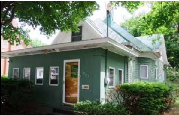
This UniverCity program home is one of 56 homes renovated by the City for owner-occupied housing .
