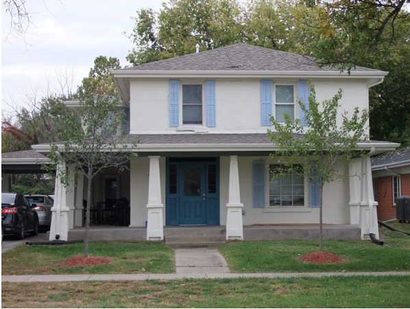
In order to address the need for African American housing, the Tate Arms building, located at 914 S. Dubuque Street, was established around 1940 and served as a private rooming house for male African American students until the mid-1960s. It was named after its owners, Junious (“Bud”) and Elizabeth (“Betty”) Crawford Tate.
