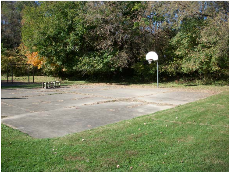
Basketball courts – lacks accessible route; plugged drain
