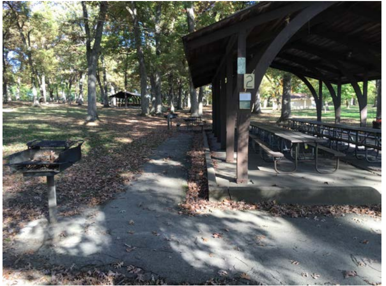
Picnic shelter – concrete in poor shape
