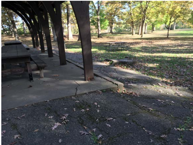
Picnic shelter – uneven surface
