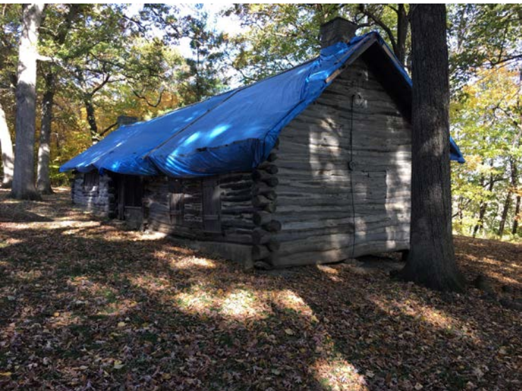
Learning center – replica log cabins in poor shape
