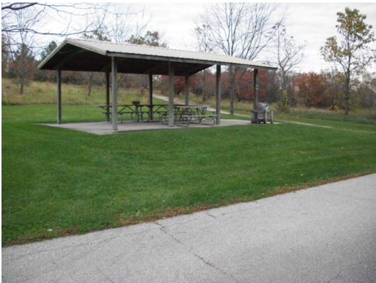
Picnic shelter – lacks accessible route
