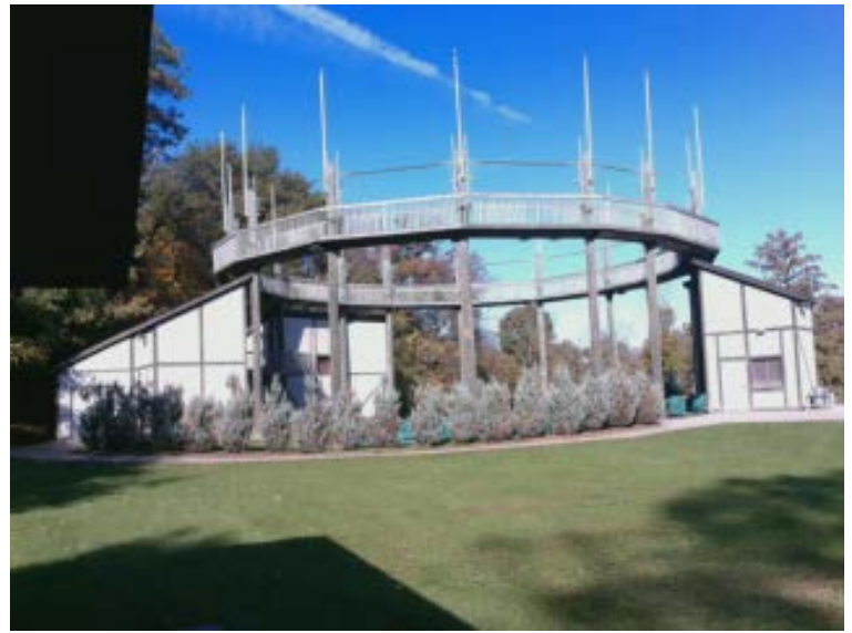
Pavilion – lacks accessible restrooms
