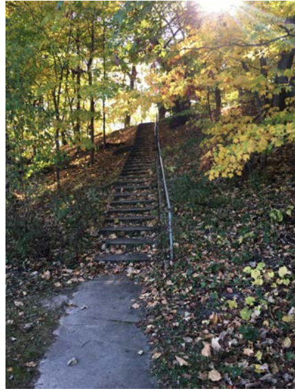
Pathway – stairs are too steep and lack handrail, poor cond.
