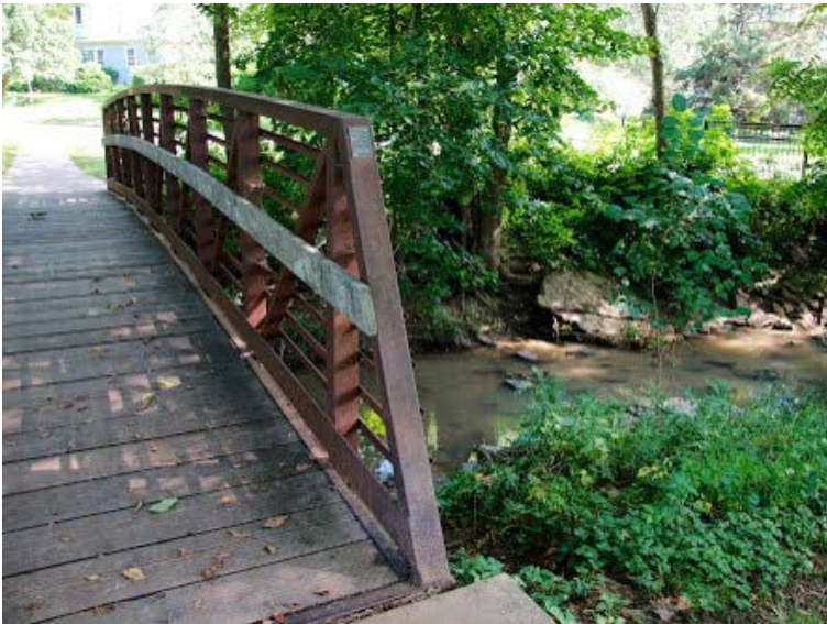
Bridge – currently being evaluated by City
