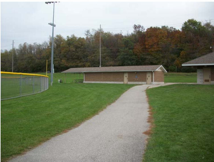
South restroom – lacks accessible fixtures
