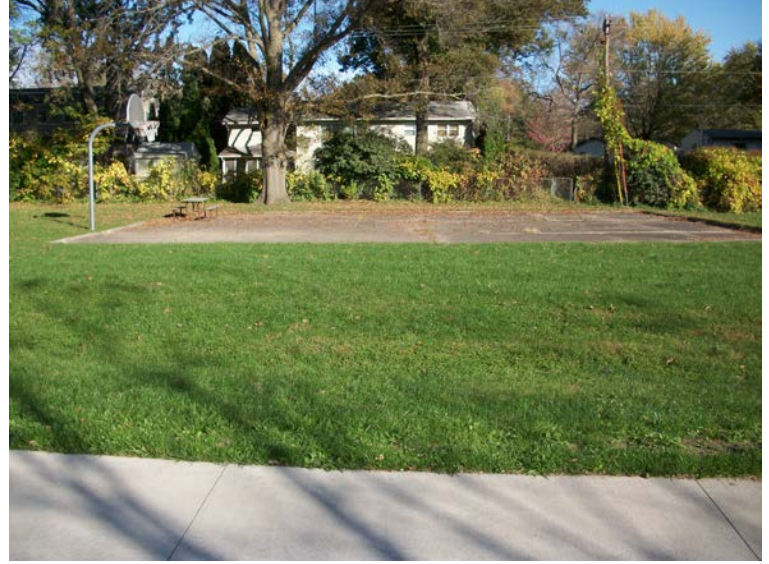
Basketball court – lacks accessible route
