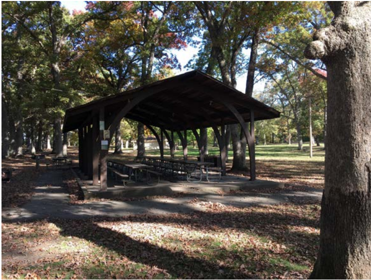
Picnic shelter – lacks ADA seating
