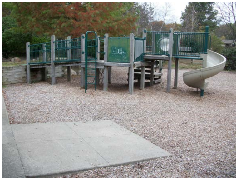
Play equipment – lacks accessible route and safety surface
