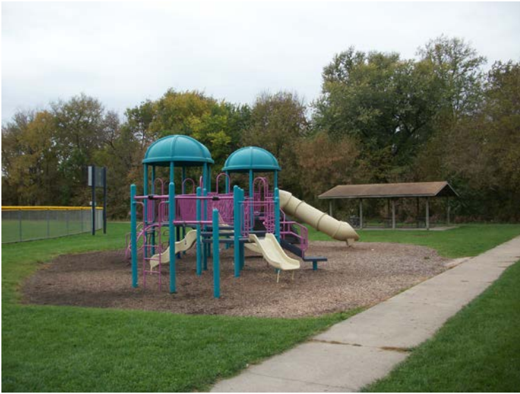
South play equip. – lacks accessible route and safety surface
