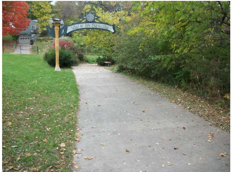
Pathway – steep slope and lacks handrails
