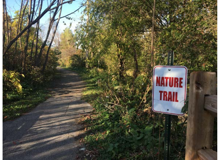
Pathway – Transition from crushed aggregate to asphalt
