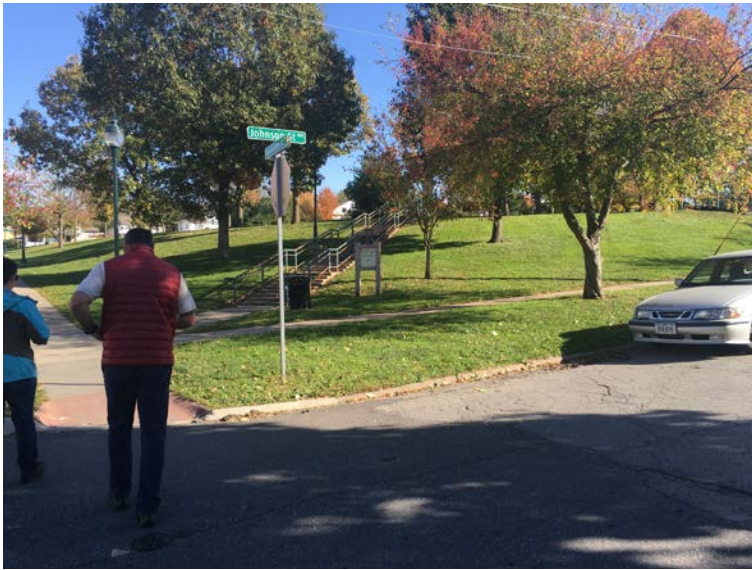
Accessible curb cut, no truncated domes
