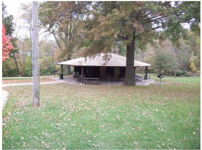
Picnic shelter – lacks accessible restroom components
