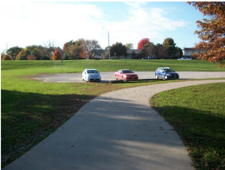
Parking – lacks accessible and designated parking
