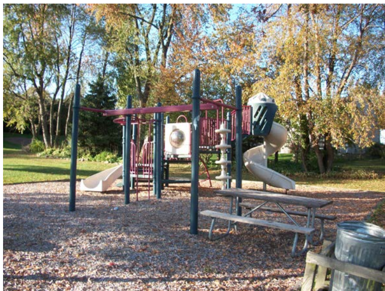
Play equipment – lacks safety surface
