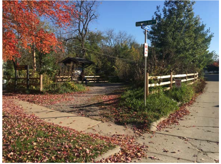
Pathway – Path is a crushed stone and is in fair to good condition
