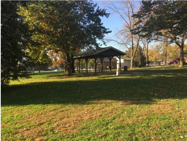
Shelter – good access to structure
