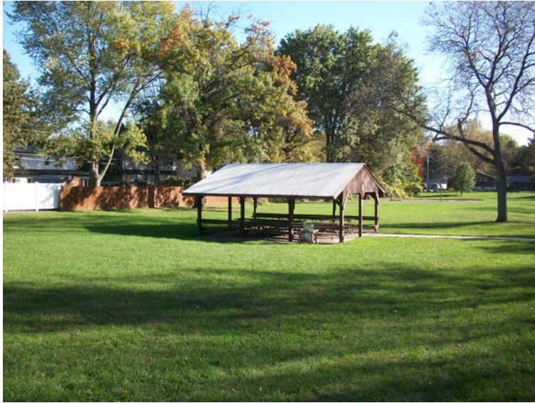
Picnic shelter – lacks accessible route
