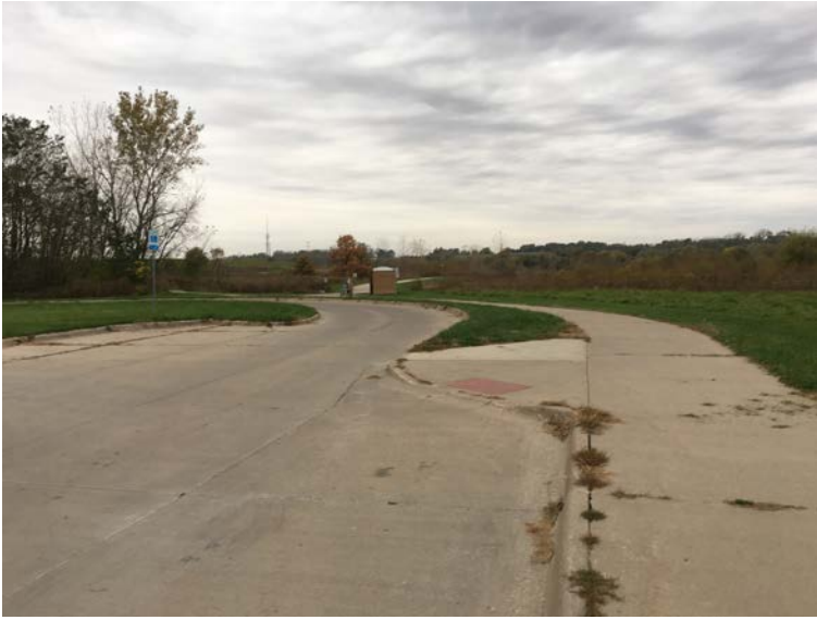
Park Identification Sign – Needs upgrading
