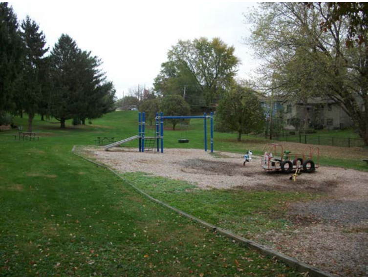
Playground – resilient surface – needs replaced
