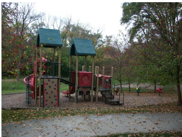
Play equipment – condition of safety surface
