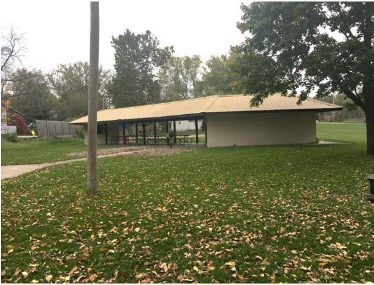
Shelter – scheduled to be replaced
