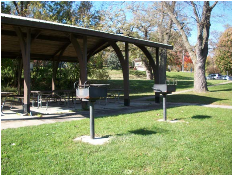
Picnic shelter south end
