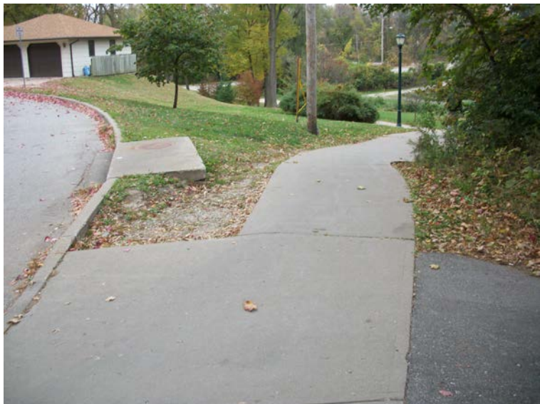
Pathway – steep slope and lacks handrails
