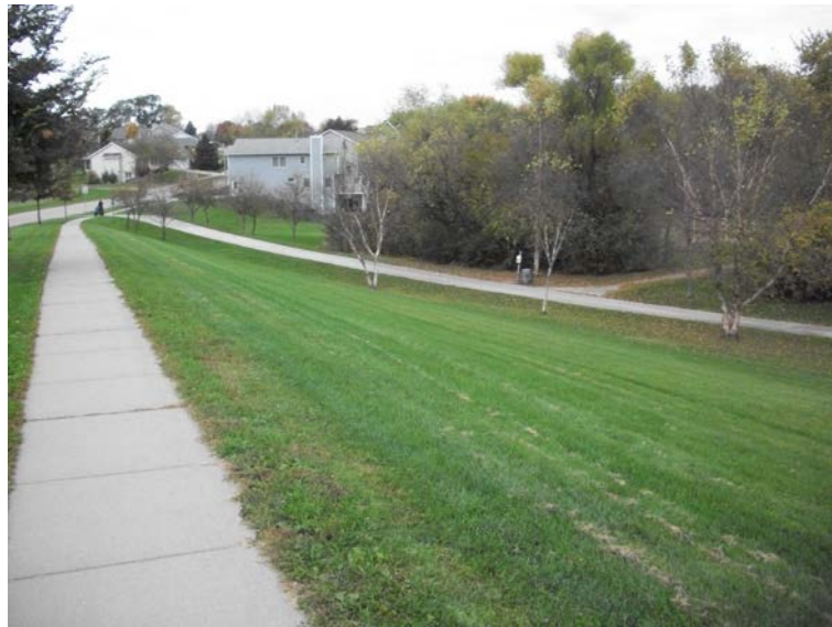
Pathway – slope exceeds 5%
