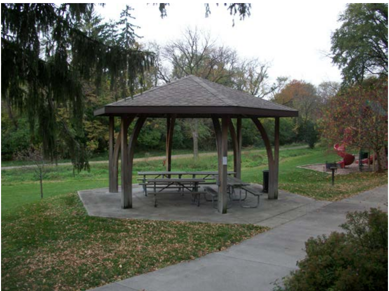
Picnic shelter – lacks accessible route
