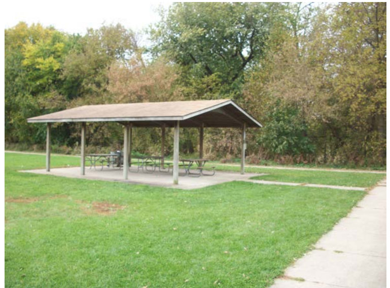
South picnic shelter
