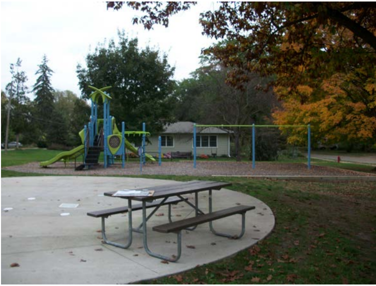
Play equipment – lacks accessible route and safety surface
