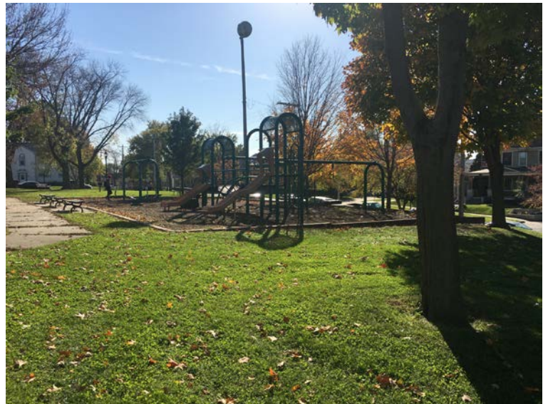
Playground – no accessible route – wood curb prohibits access
