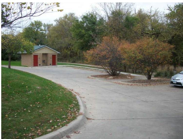
Parking – lacks accessible and designated parking
