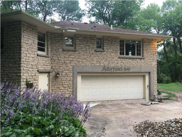
Back property under construction
