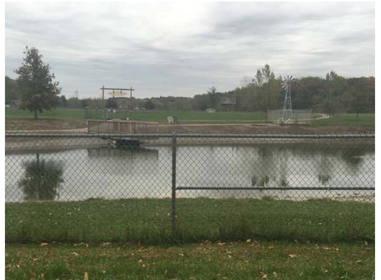
Access – Interior access to pond and pier.
