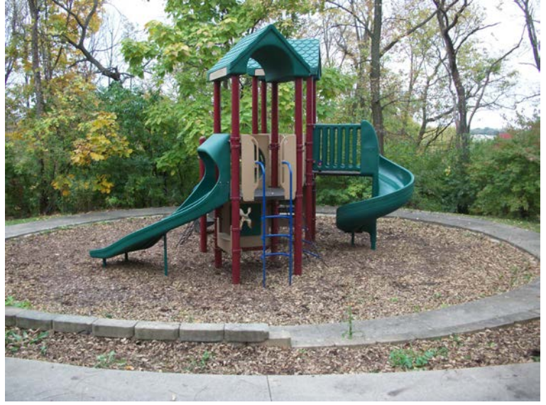
Play equipment – lacks safety surface
