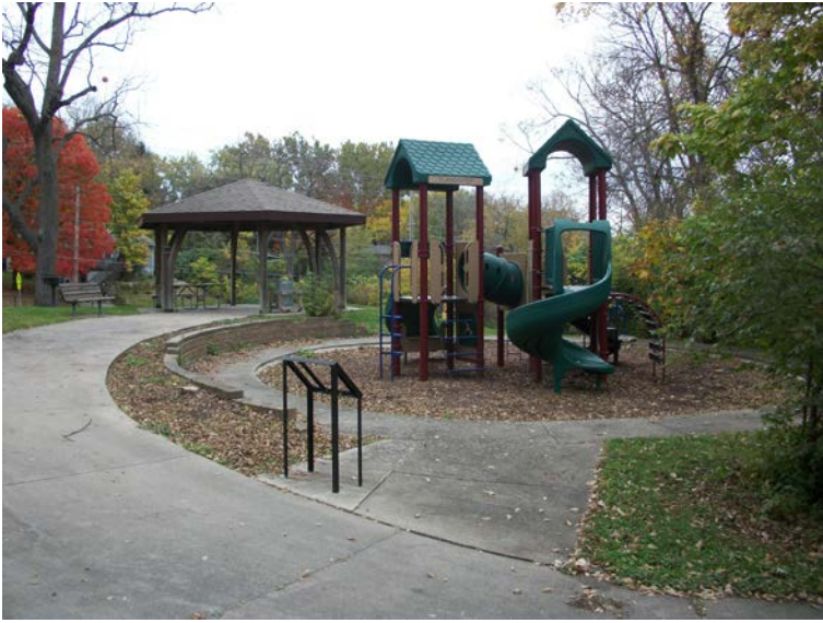
Play equipment – lacks accessible route (due to pathway)
