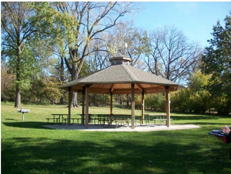
Picnic shelter – lacks accessible route
