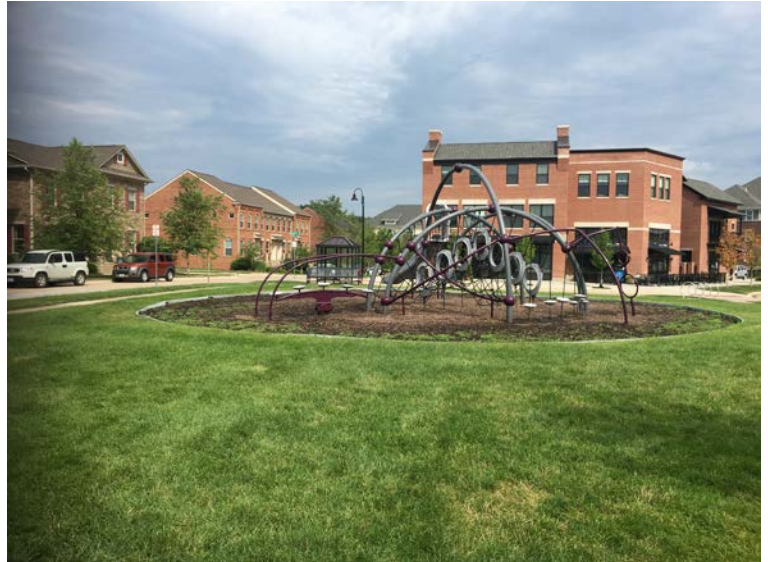
Playground – no pathways to playground
