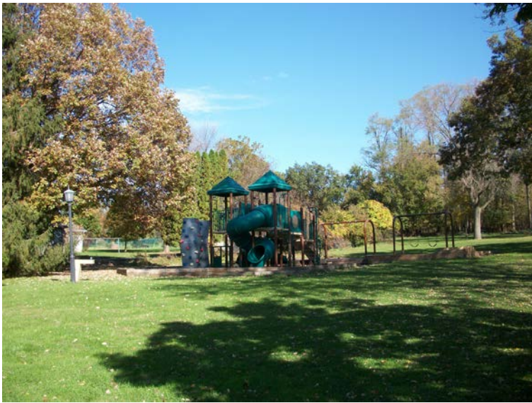
Play equipment – lacks accessible route
