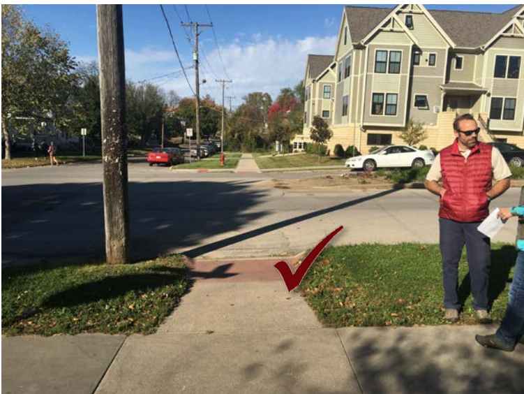
Accessible routes – curb cuts – no truncated domes
