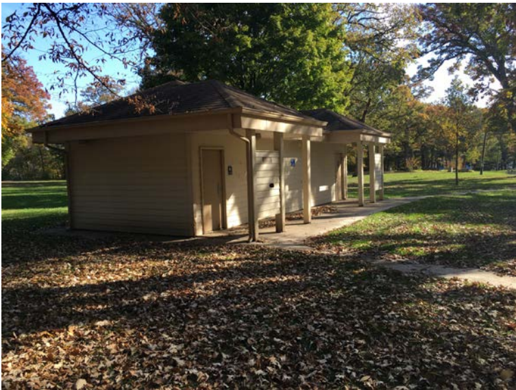
Restroom – needs painting
