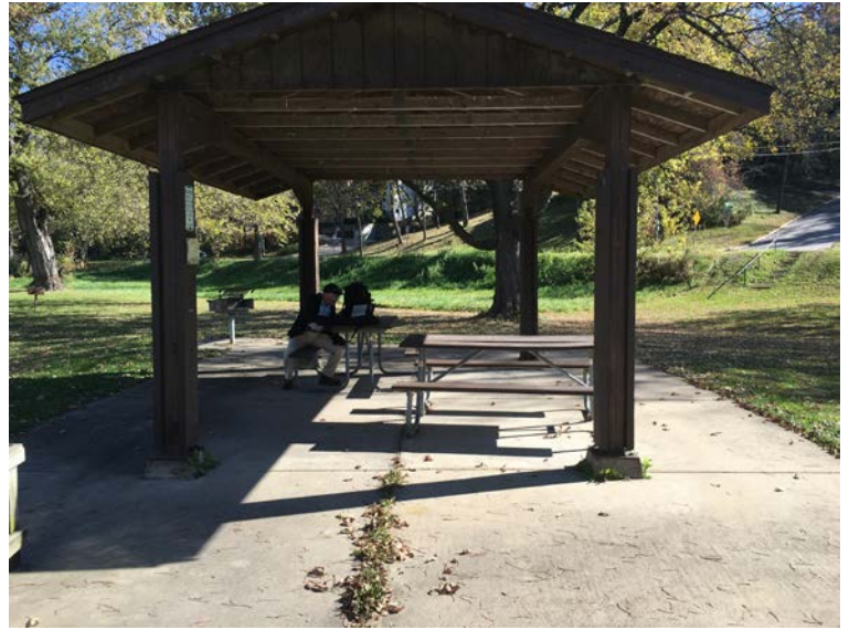
Picnic shelter – lacks accessible tables
