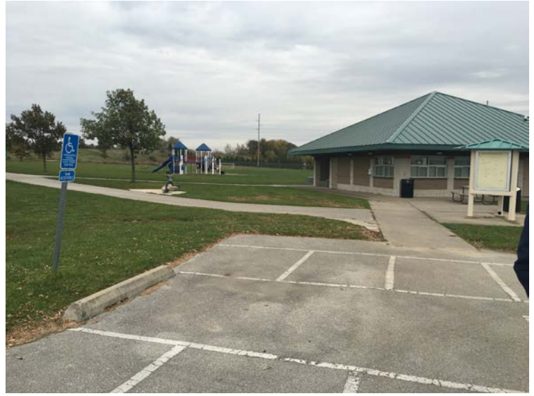
Access – Good interior access to main structures
