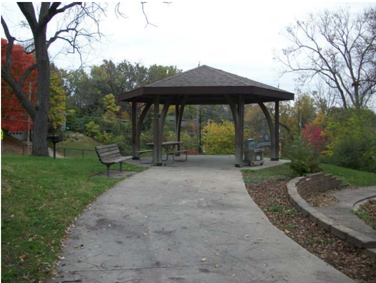
Picnic shelter – needs new stain coat
