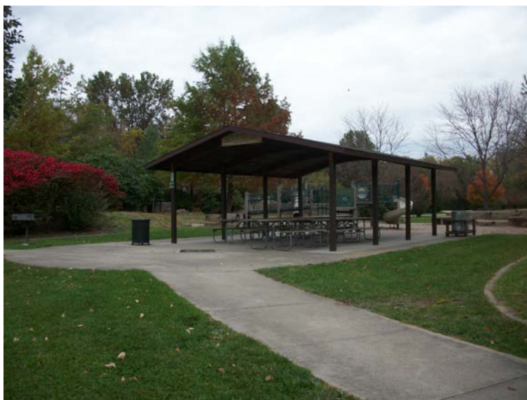
Picnic shelter – lacks accessible table
