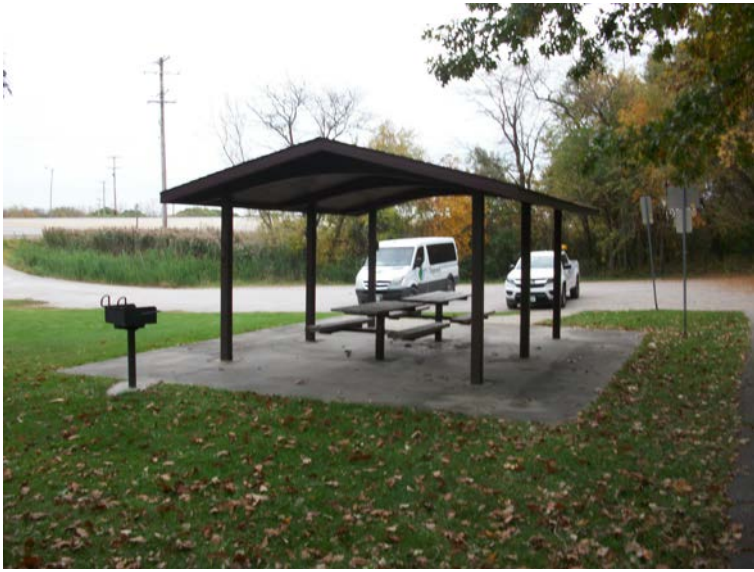
Picnic shelter – lacks accessible table
