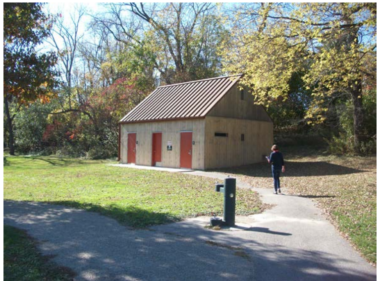
Restroom south end
