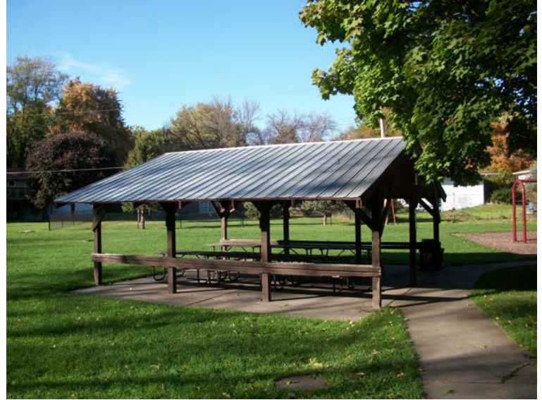
Picnic shelter – lacks accessible route
