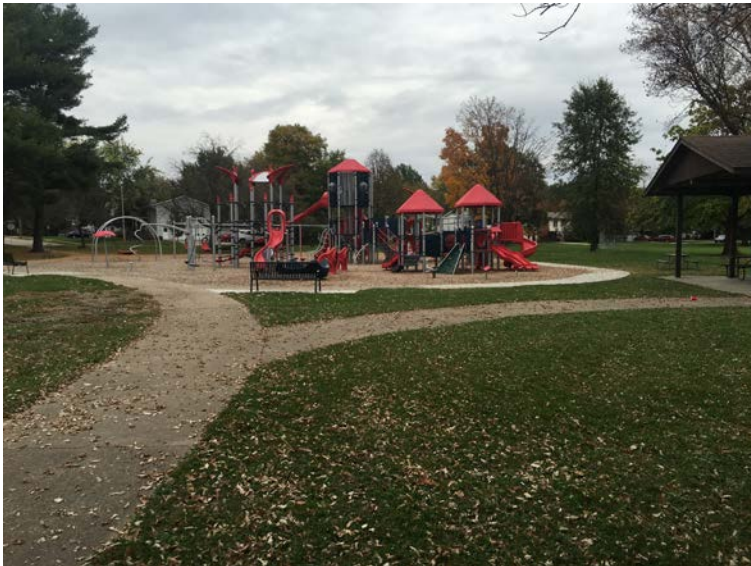
Access – Good access to play structure and adjacent facilities
