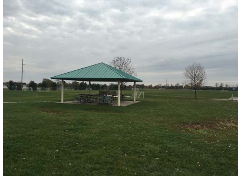
Access – limited interior access to shade structures
