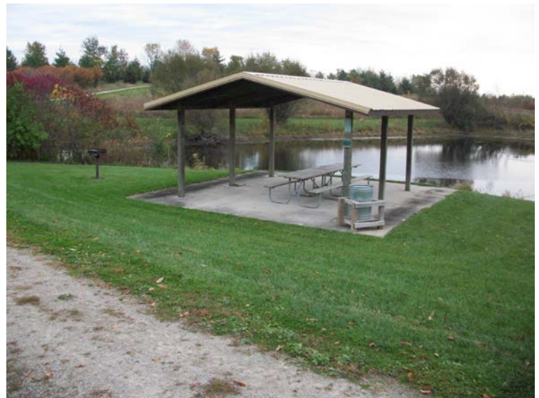
Picnic shelter – lacks accessible route
