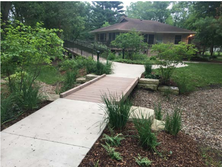
Pathway & Ramp to House – good access to adjacent areas
