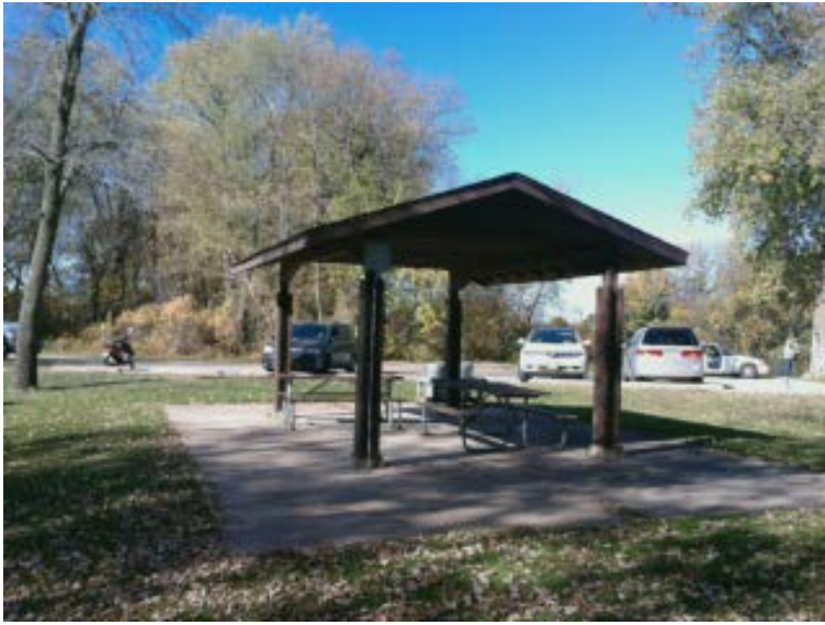
Picnic shelter– lacks accessible route
