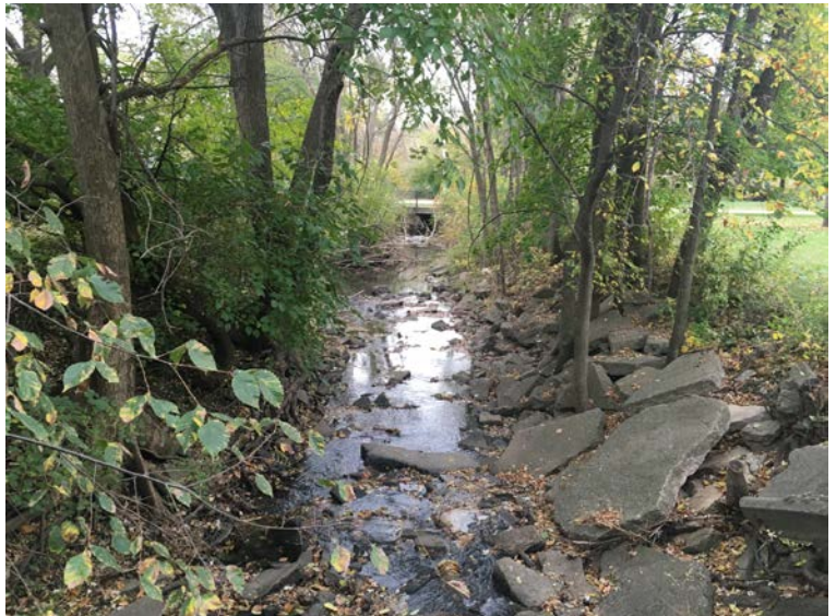
Creek Access – opportunity for creek access
