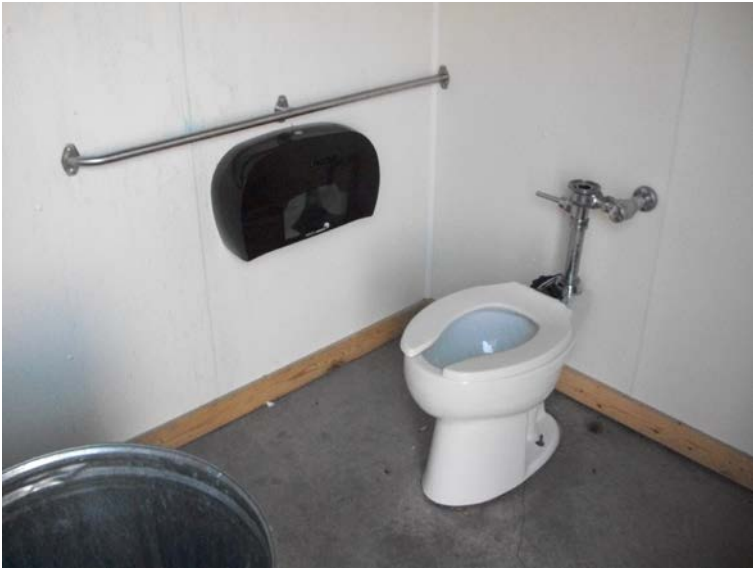
Restroom north end – lacks accessible fixtures
