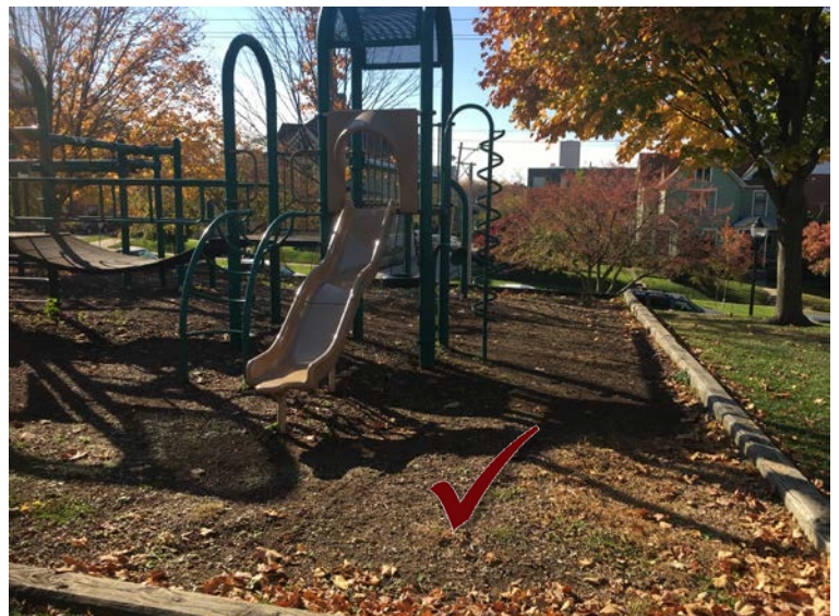
Playground – resilient surface – needs replaced
