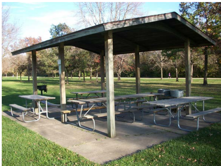
Picnic shelter – lacks accessible route to accessible table
