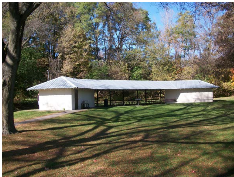
Picnic shelter – poor condition
