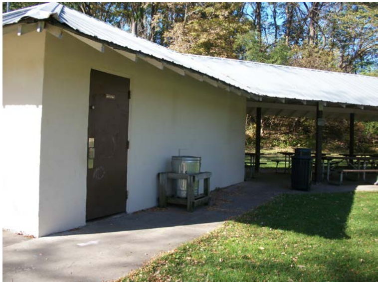
Restrooms – lack accessible fixtures
