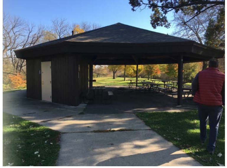
Picnic shelter north end – lacks accessible tables
