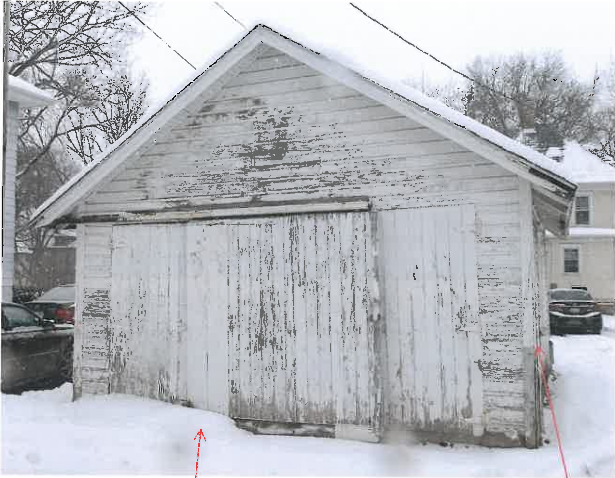
sliding door with hinged doors on each side
