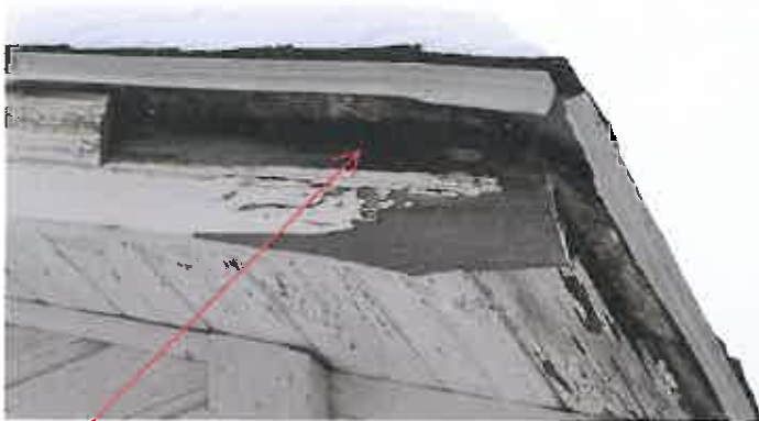
rotten roof material under shingles
