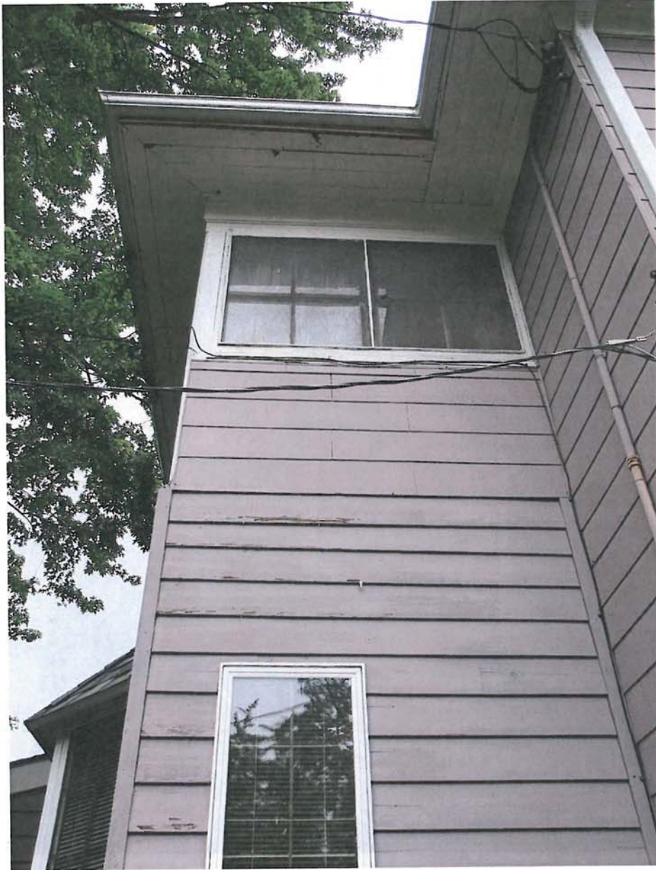
1154 Court Street detail of west side sleeping porch windows
