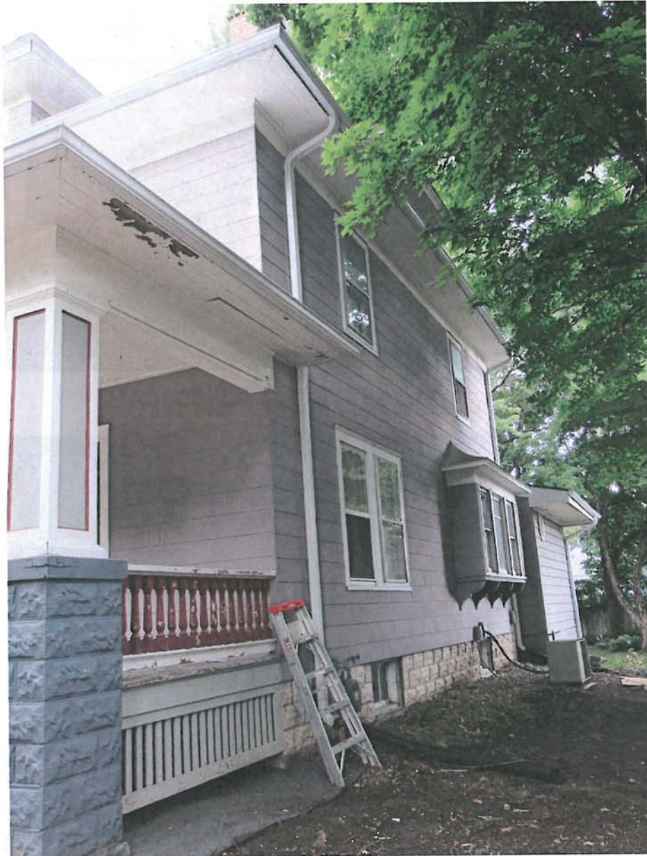
1154 Court Street- side detail showing historic projecting bay and 1960s addition behind. Original block porch pier in the foreground matches unpainted foundation wall.
