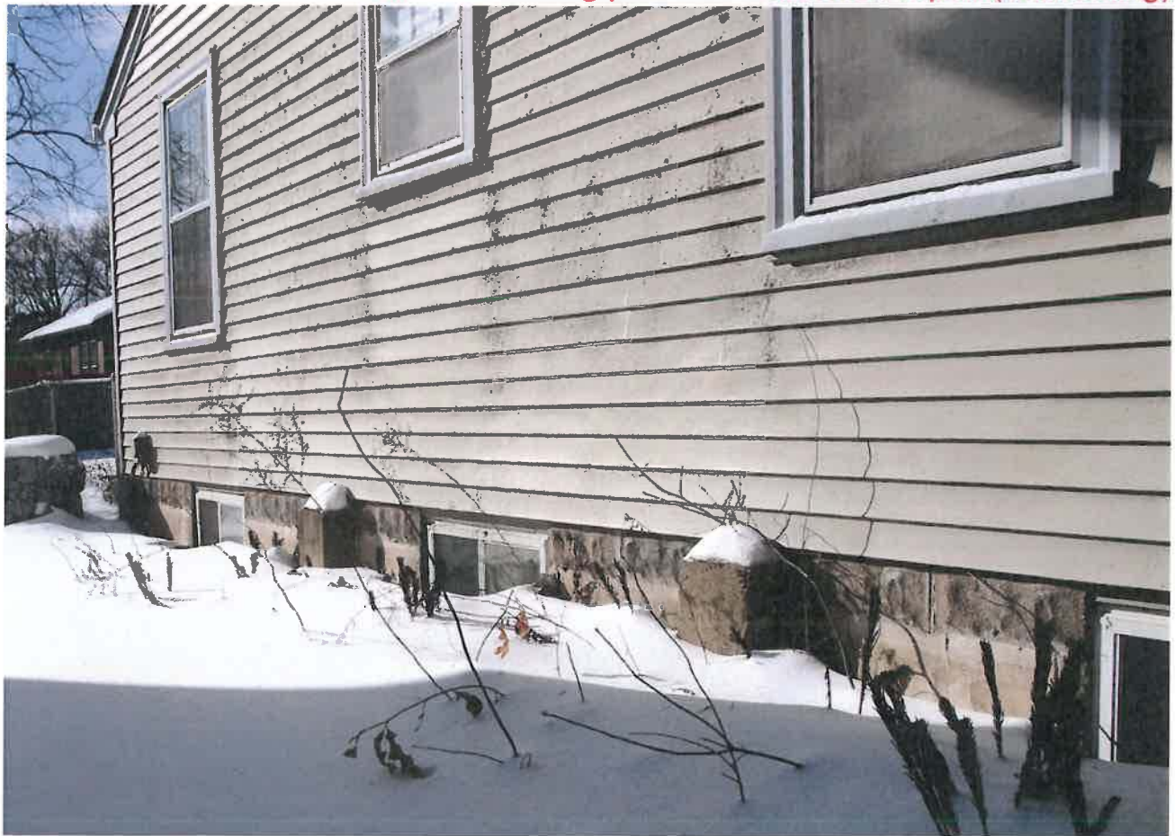
house east side showing previous foundation repair (buttressing)
