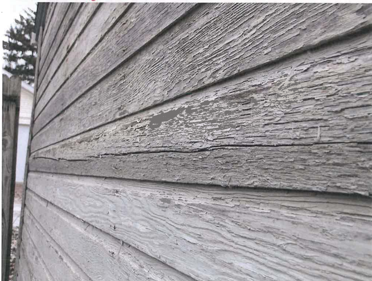
Deteriorated siding detail
