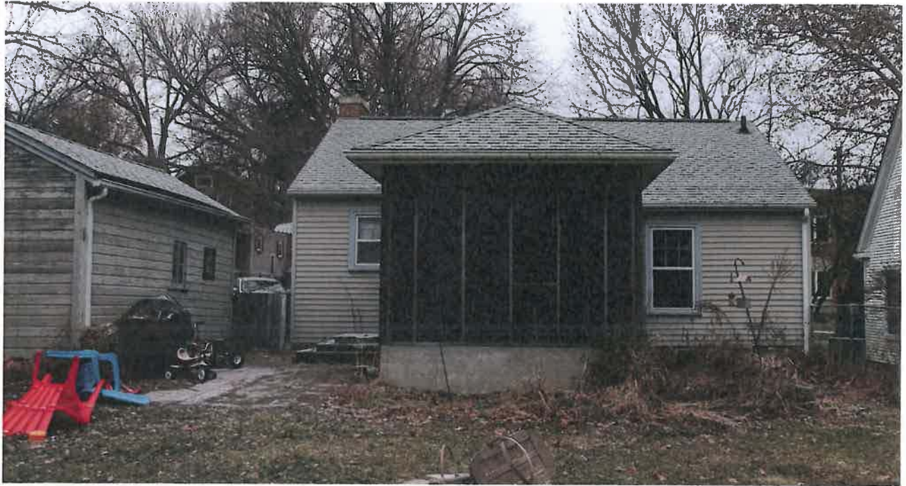
house east side showing previous foundation repair (buttressing)
