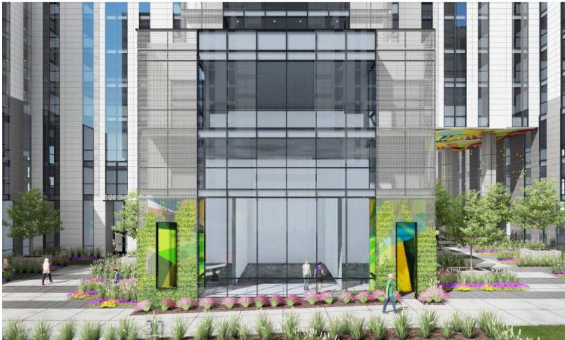
Figure 4. Metal Panels with Graphic Panels along Capital Street
