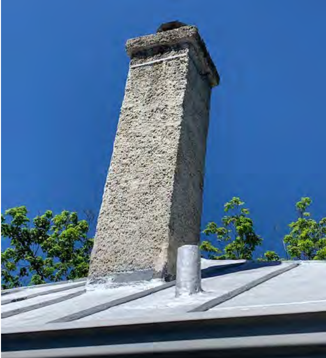
Detail of chimney
