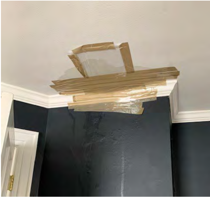
Interior damage from chimney
