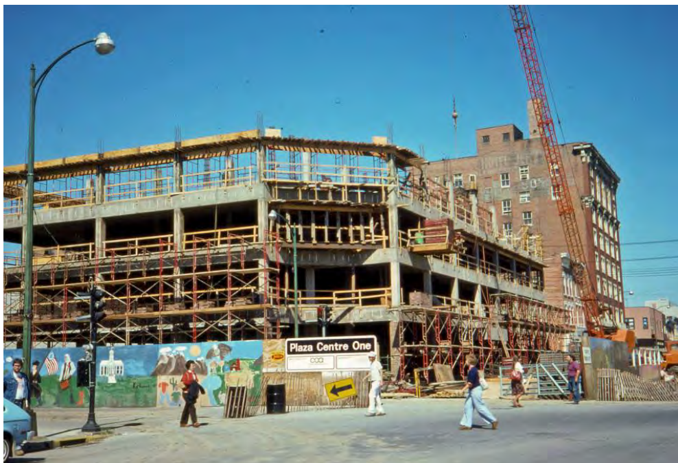
Figure 12. Plaza Centre One Under Construction – Spring, 1978
