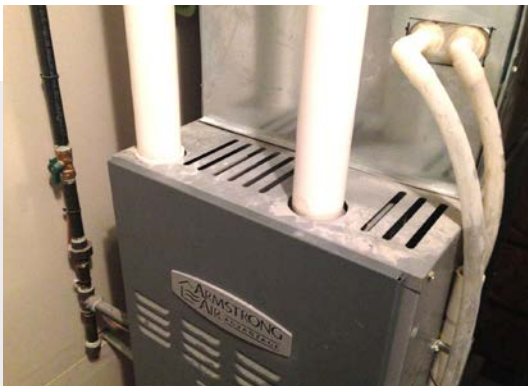
A high-efficiency furnace includes a sealed combustion area that uses PVC piping for air intake and exhaust as shown in this photo.
