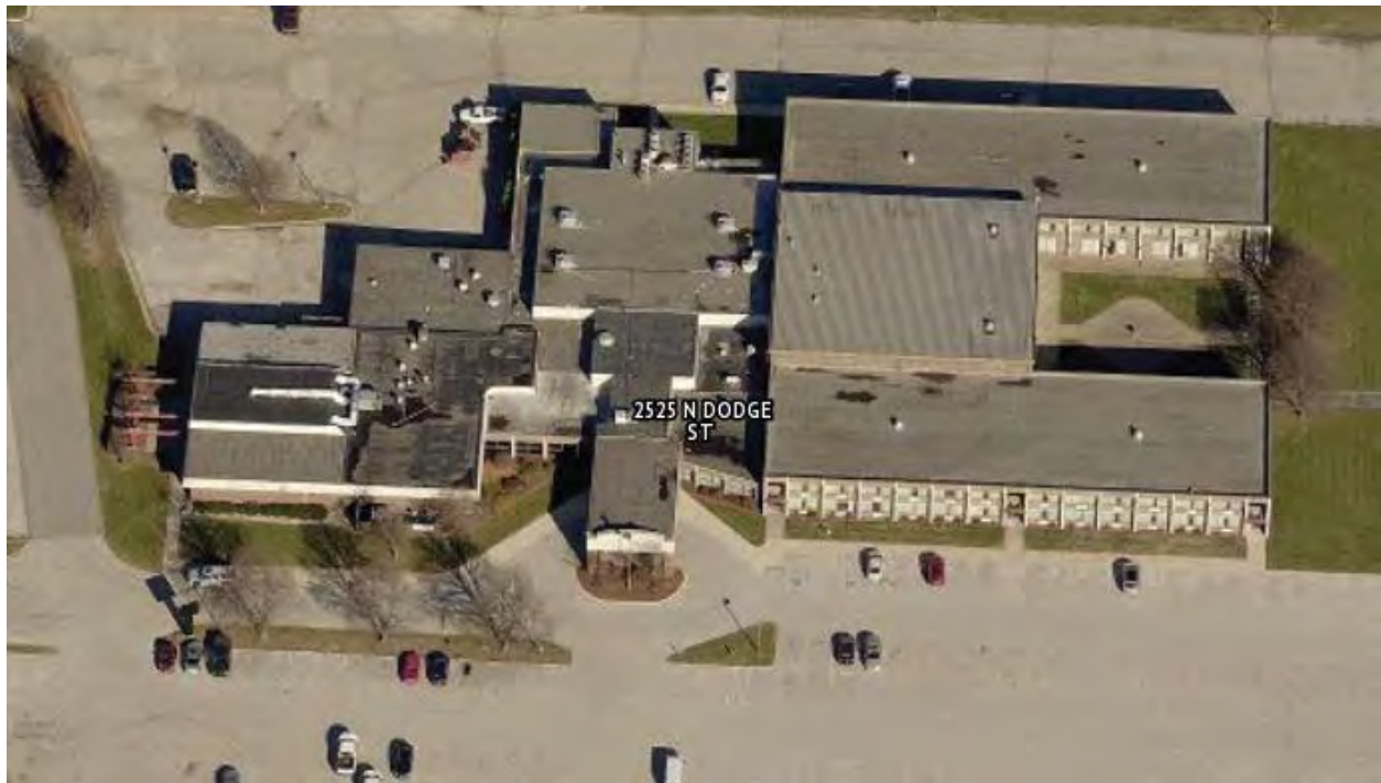
Figure 7-2: Rooftop view of the building looking north (Johnson County Assessor, 2020) (note that the west canopy beams are still in place, pergola-like)
