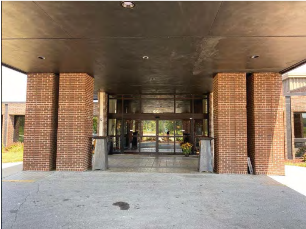
Photo Number 7: Description: Motel addition, south entrance detail, looking north
