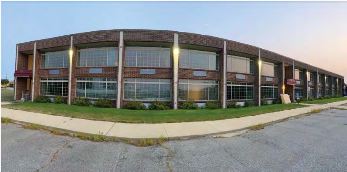
Photo Number 13: Description: Motel addition, north wing, looking south
