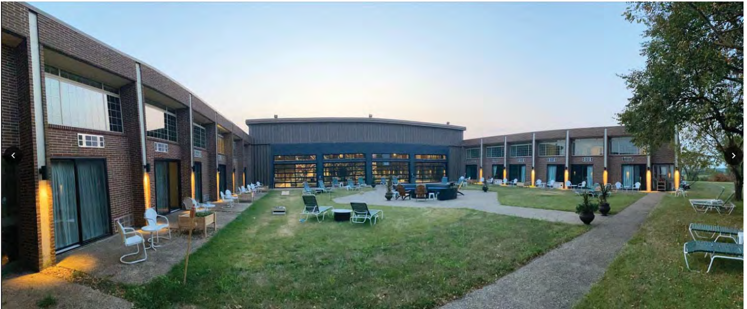
Photo Number 12: Description: Motel addition, courtyard, looking northwest
