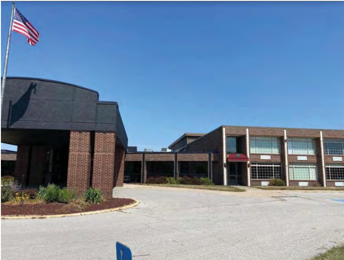
Photo Number 8: Description Motel addition, south entrance and offices, looking north:
