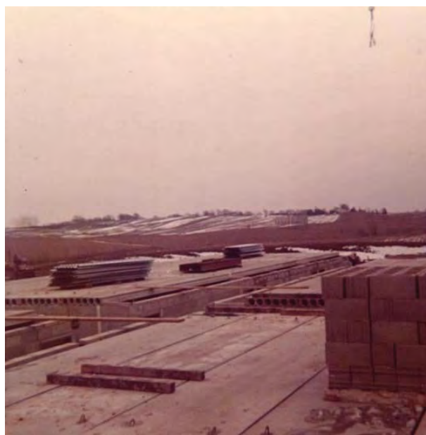
Figure 8-44: Construction photos, lower level of south motel wing decked, looking northeast, both December 1972 (Courtesy of Sheila Boyd)
