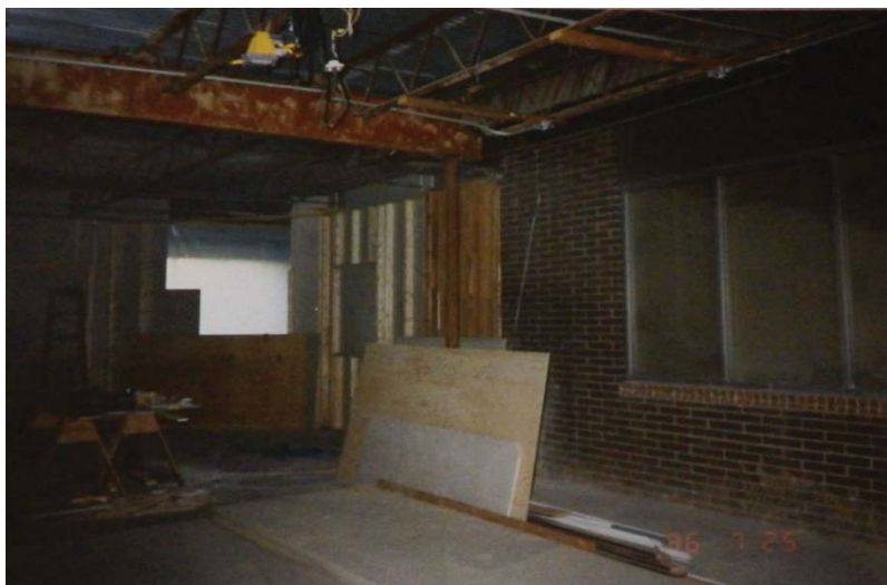
Figure 9-115: Interior view showing former supper club exterior window, looking southwest, 1996 (owner scrapbook)
