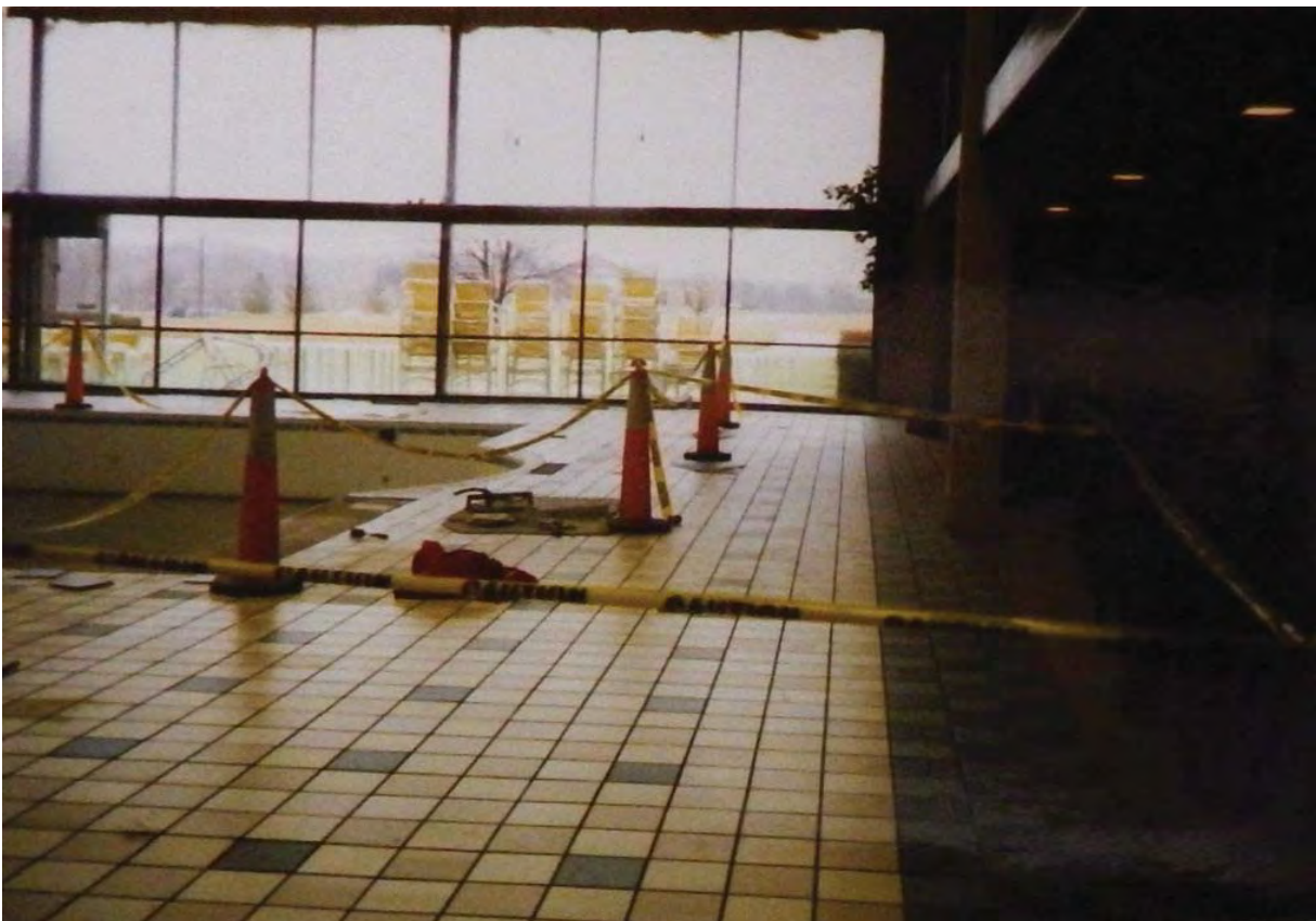
Figure 8-107: Tiled floor installed in the pool court, 1984, looking east (owner scrapbook)
