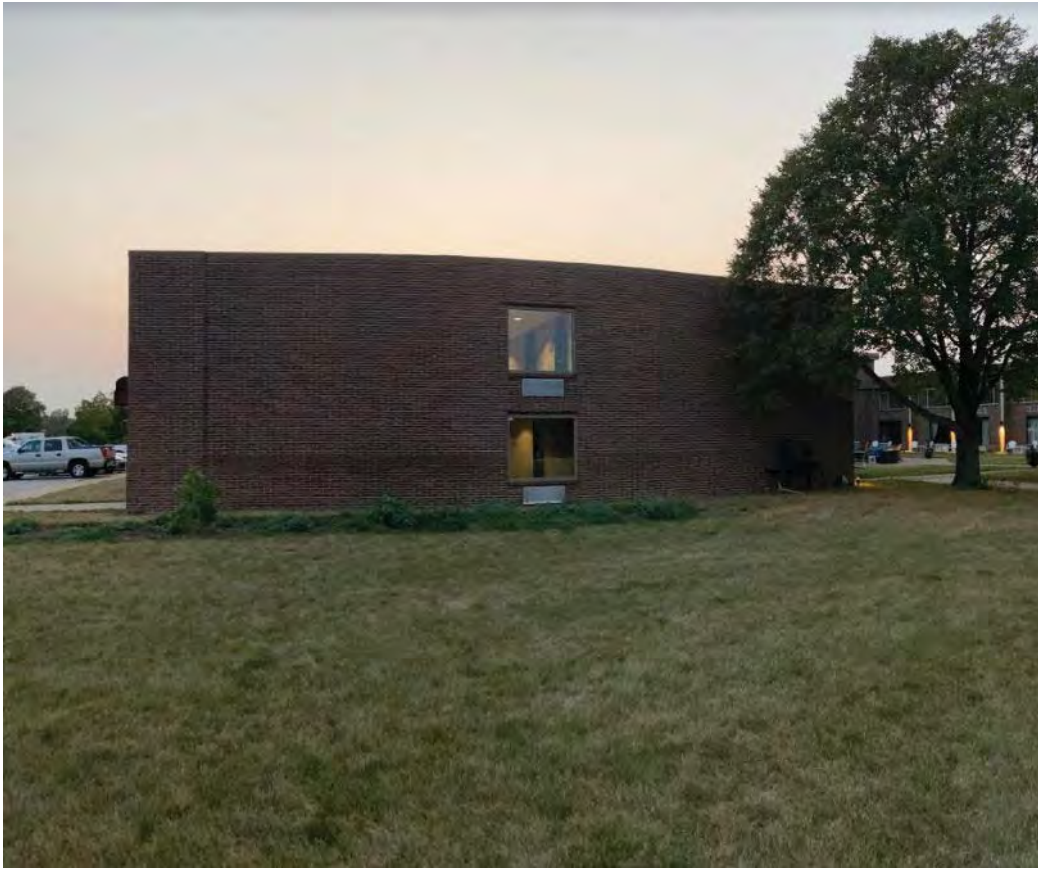
Photo Number 11: Description: Motel addition, east end wall of the south wing, looking west
