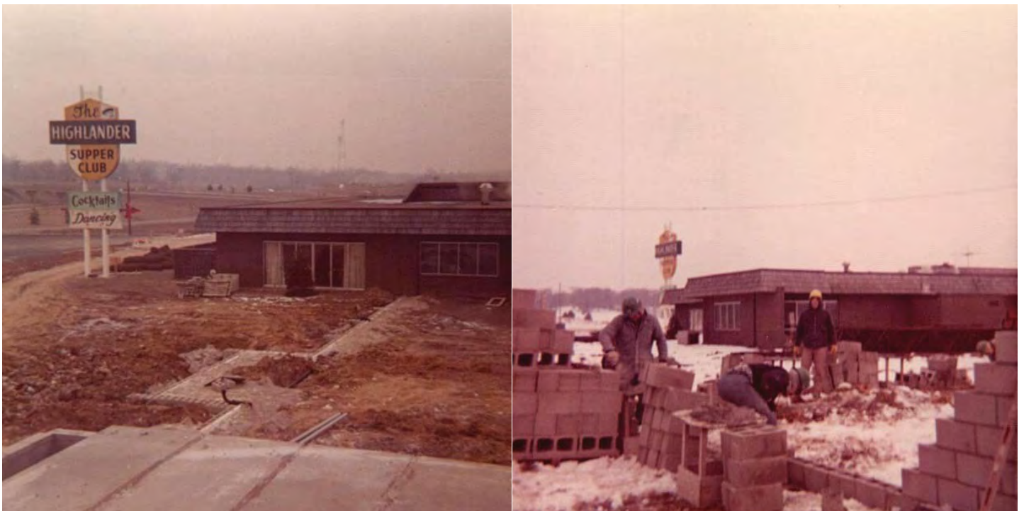
Figures 8-40, 8-41: Construction photos; Left, looking west, supper club and sign, note footings and new south entry, right, supper club original north wall looking southwest, both December 1972 (Courtesy of Sheila Boyd)
