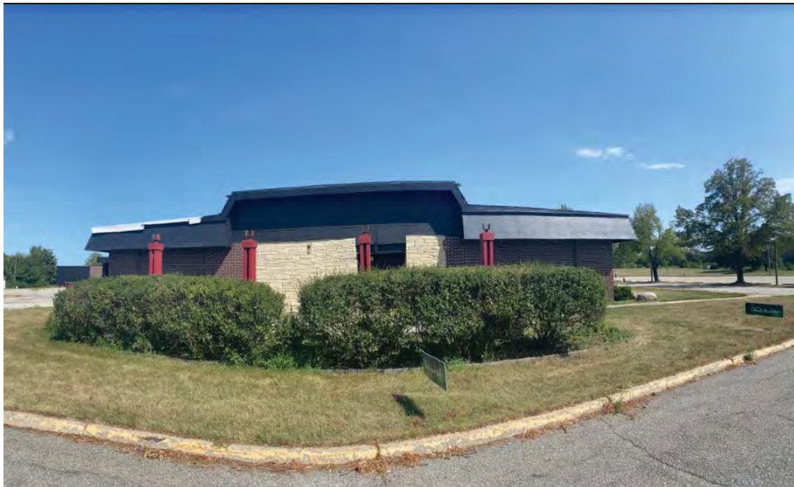
Photo Number 2: Description: Supper club entrance looking east, note support pillars for porte cochere
