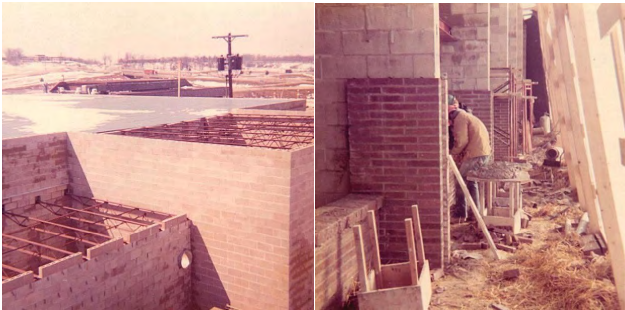
Figures 8-47, 8-48: Construction photos, left, roof framing and wall details, looking west, and right, veneer work on south motel wing, south facade, looking east, both May 1973 (Courtesy of Sheila Boyd)
