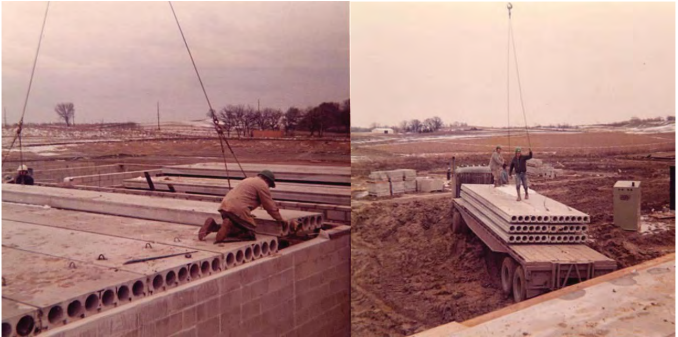
Figures 8-42, 8-43: Construction photos; Left, looking northeast, precast hollow floor panels, right, load of panels, looking northeast, both December 1972 (Courtesy of Sheila Boyd)
