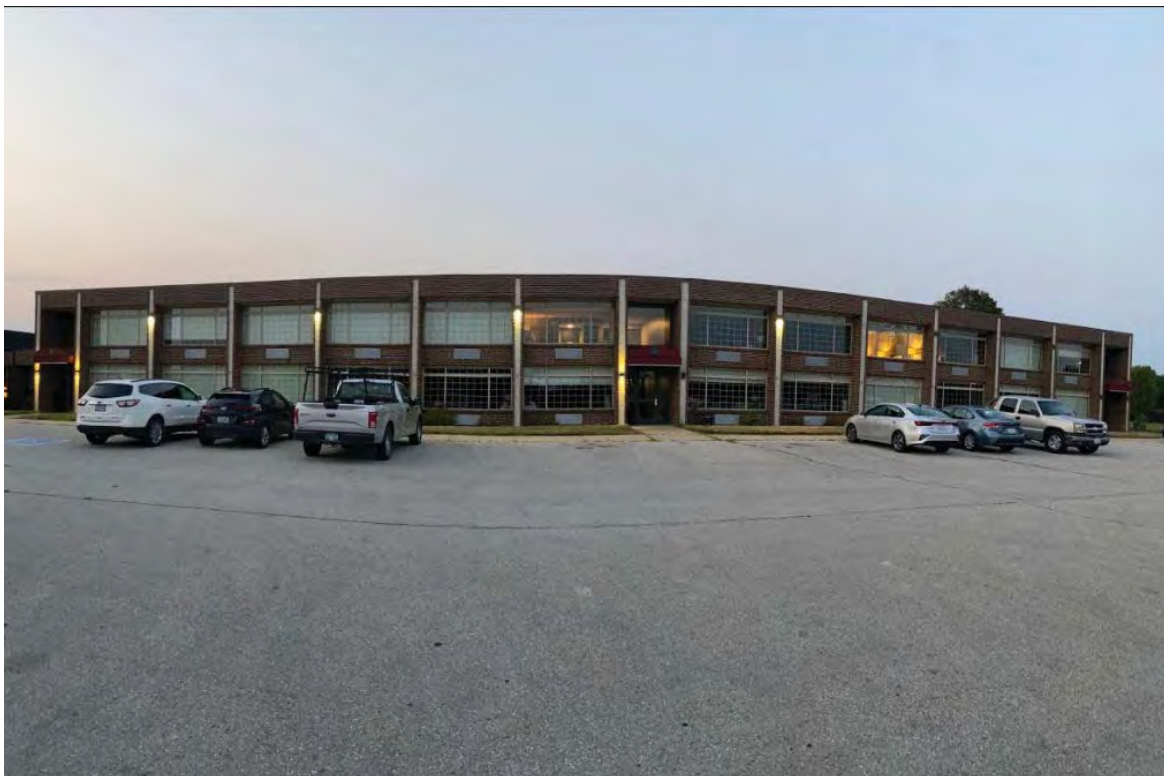
Photo Number 10: Description: Motel addition, south wing, looking north
