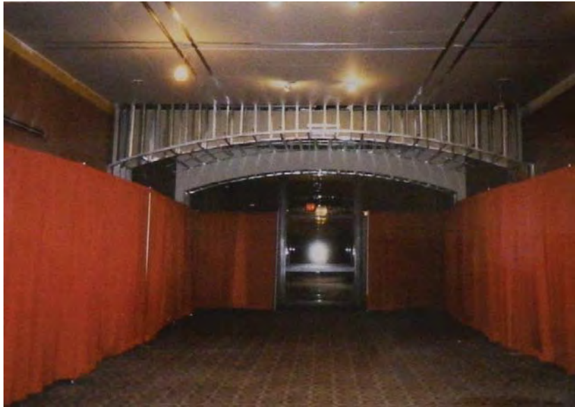
Figure 8-113: Constructing arches in main hallway, looking north (owner scrapbook)
