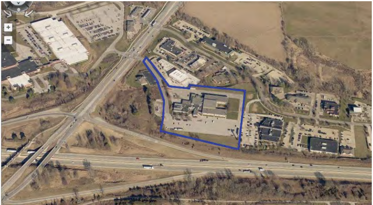
Figure 10-3: Assessor's aerial photo with property line overlay, looking northwest (Johnson County Assessor, 2020)
