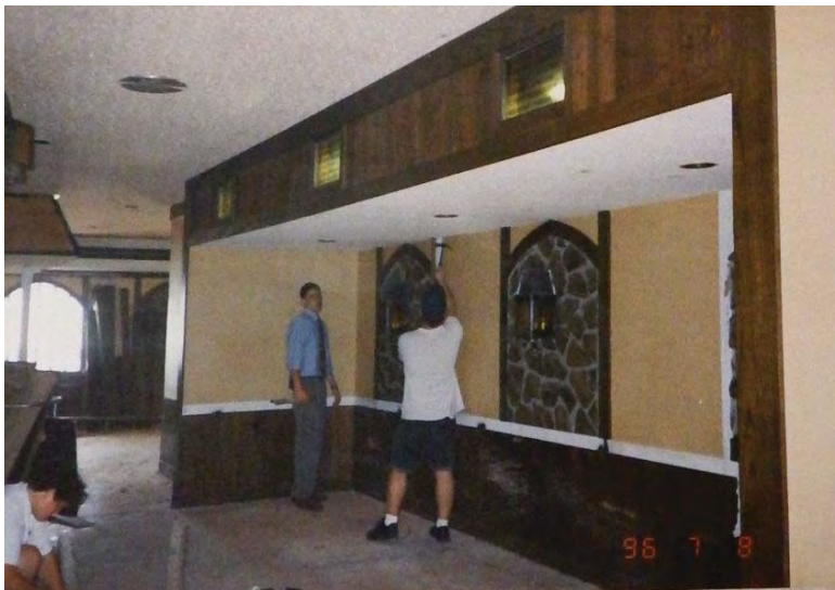
Figure 8-111: Former Royal Scot Dining room, note faux mansard, pointed arch windows with stone infill, stained glass, wainscot, 1996, looking south (owner scrapbook)
