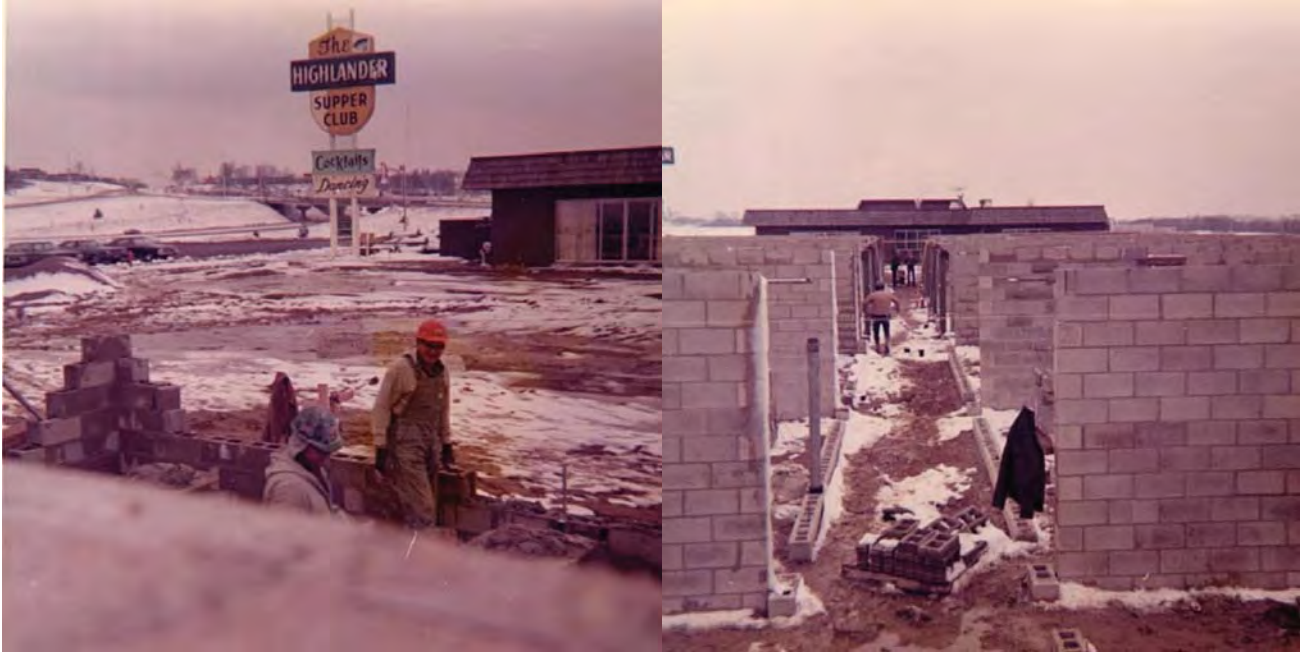
Figures 8-38, 8-39: Construction photos; Left, looking southwest, supper club and sign, right, south motel wing looking west, both November 1972 (Courtesy of Sheila Boyd)
