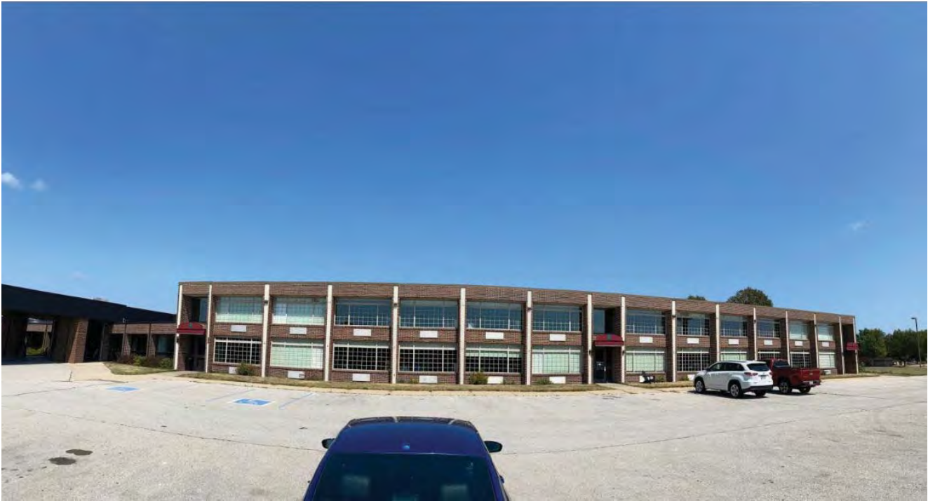
Photo Number 9: Description: Motel addition, south wing, looking north
