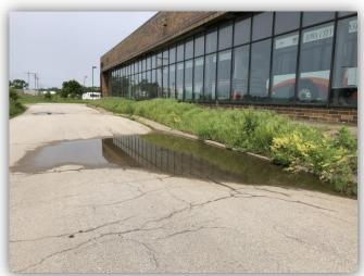
Asphalt patching, persistent ponding of water, wetland formation, potholes, uneven surfaces are common and cause hazards for vehicles and pedestrians.
