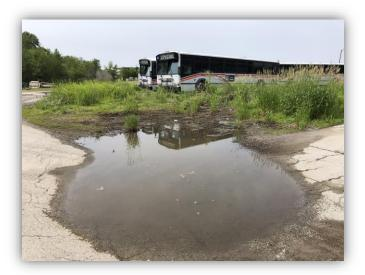
Annual asphalt patching required to ensure buses have an adequate slope to enter/exit the building.
