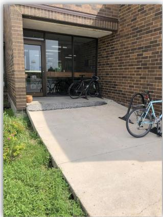
The once-level pedestrian approaches are now considerably sloped, are no longer ADA compliant, and require asphalt patching.
