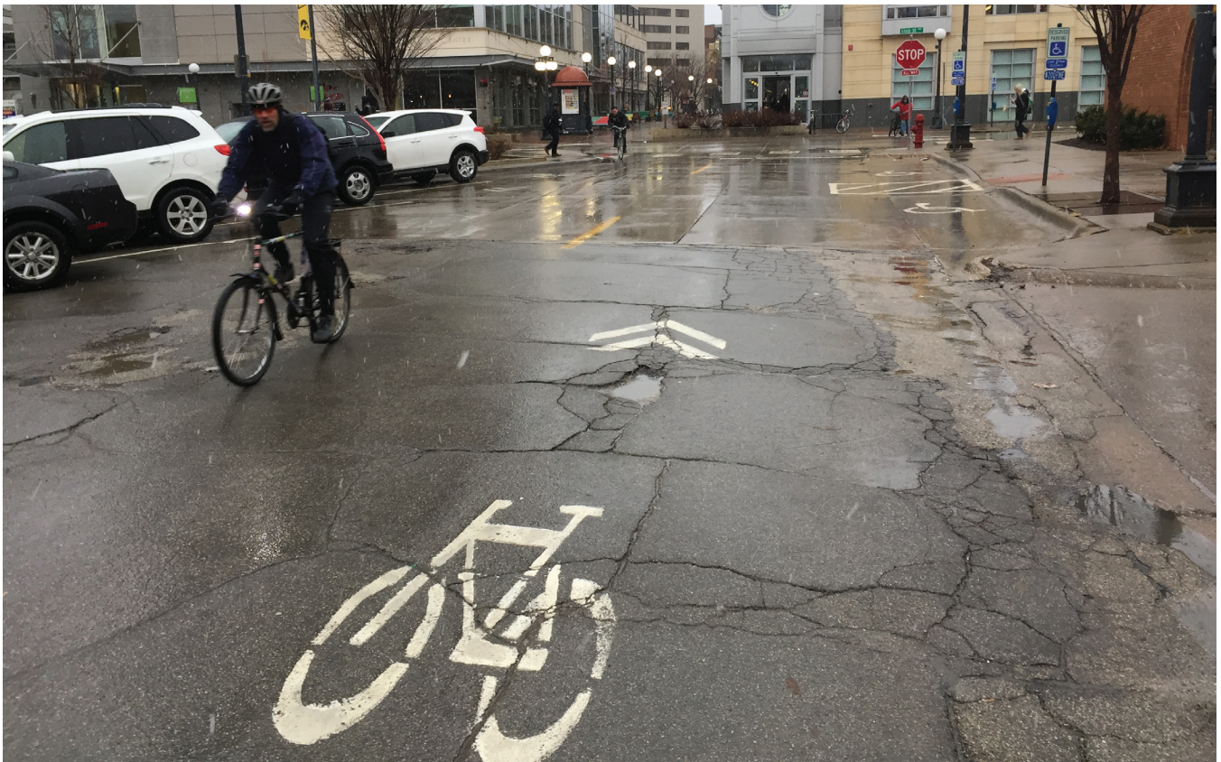
Figure 8. Cracks, debris and potholes like the one seen here on College Street represent significant hazards to bicyclists.
