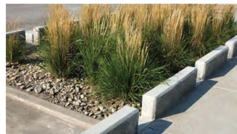
The bioretention planting areas will collect, cleanse, slow, and infiltrate storm water.
