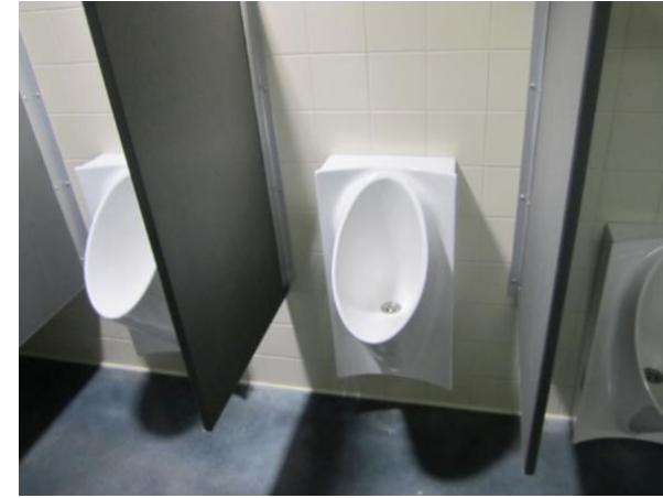
Low-flow and automatic fixtures
