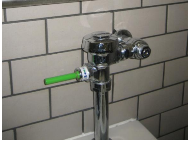
Dual volume flush toilet
