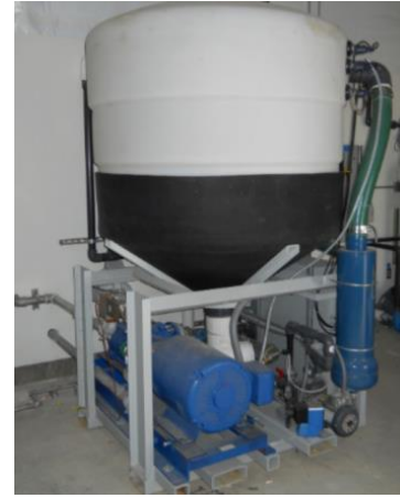
Wash water reclaim system
