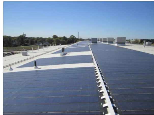
Photovoltaic panels on roof
