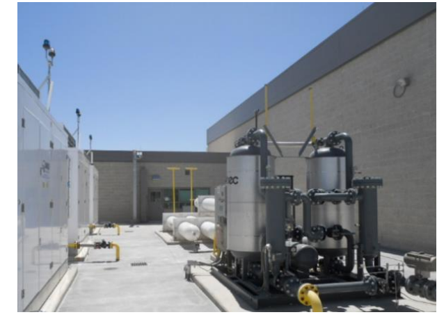
CNG fueling for buses and non-revenue vehicles
