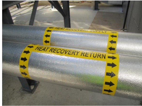
Heat recovery piping
