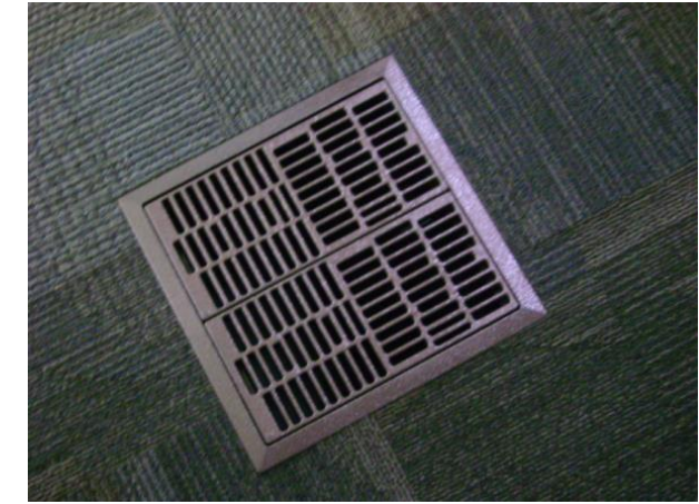
Under floor air distribution
