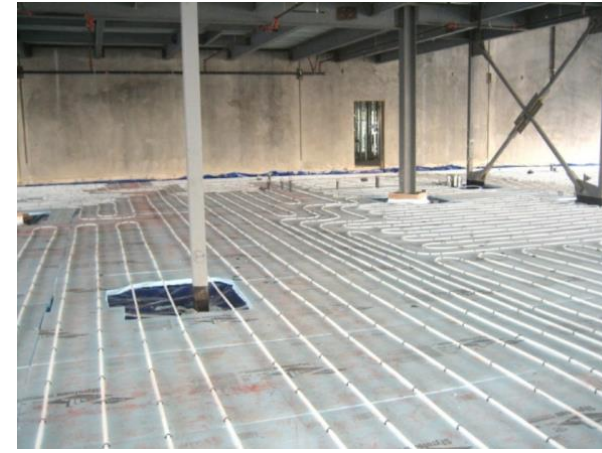
Radiant floor system
