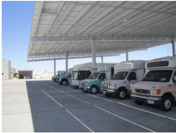
Photo-voltaic shade structure
