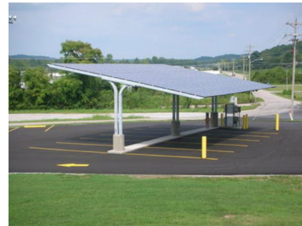
Photovoltaic panel on parking canopy
