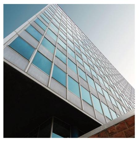
incorporate rain screens and glass fiber reinforced concrete panels (GFRC). Because curtain wall construction uses relatively light-weight and less expensive materials, it reduces building costs, which, in part, explains its popularity.
