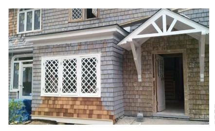
[5] Rotted wood shingles have been replaced in kind with matching wood shingles.
