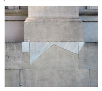
[3] **Not Recommended:** Although the Dutchman stone repair has been well executed, the replacement stone is not a good color match.
