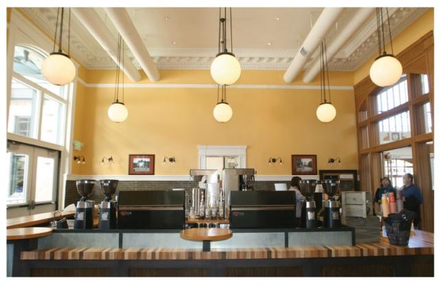
[37] Exposed and painted ducts were appropriately installed here in a retail space in Denver's historic Union Station after considering other options that would have impacted the ceiling height, or damaged or obscured the ornamental plaster crown molding. Photo: Heritage Consulting Group.
