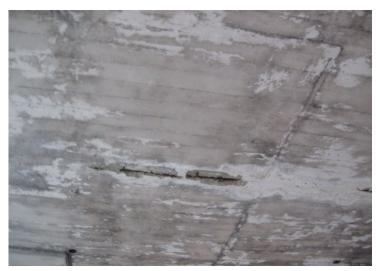
[5] Rebars in the reinforced concrete ceiling have rusted, causing the concrete to spall. The rebars must be cleaned of rust before the concrete can be patched.
