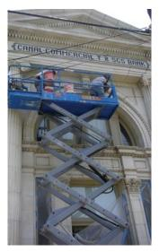
[1] An alkaline-based product is appropriate to use to clean historic marble because it will not damage the marble, which is acid sensitive.
