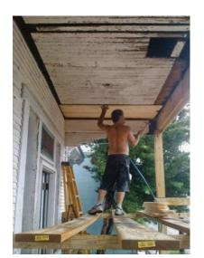
[24] Rotted boards in the beaded-board porch ceiling are being replaced with new matching beaded board.
