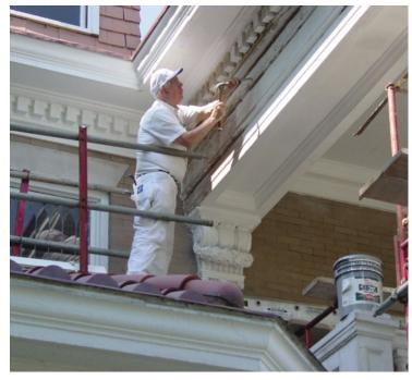
[12] Repair and limited replacement in kind to match deteriorated wood porch features is always a recommended preservation treatment.
