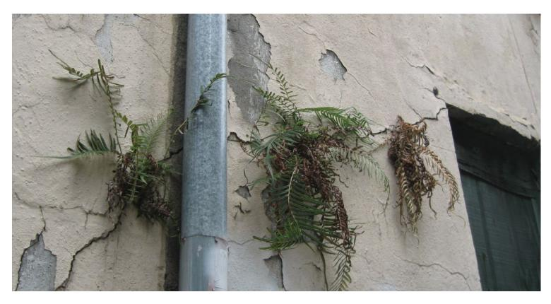
[3] **Not Recommended:** Cracks in the stucco have not been repaired, thereby allowing ferns to grow in the moist substrate which will cause further damage to the masonry.
