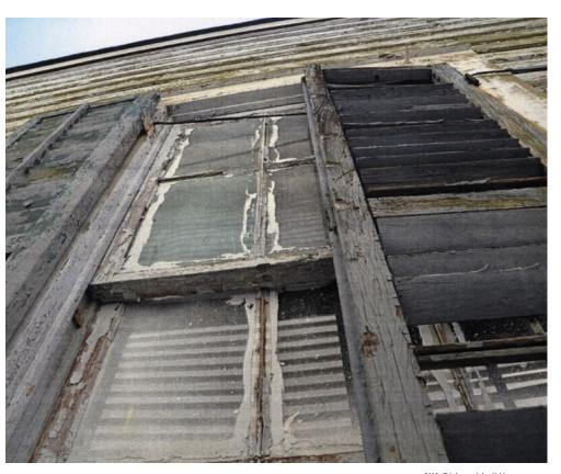
[11] Old and brittle glazing putty should be removed carefully before reputtying to keep window glazing weathertight.
