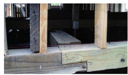
[33] Retaining as much as possible of the historic wood sill plate and replacing only the termite-damaged wood is always the preferred and recommended treatment.
