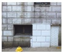
[1] A test patch should always be done before using a chemical cleaner to ensure that it will not damage historic masonry, as in this instance, terra cotta.
