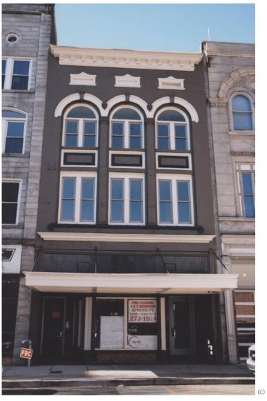
[22] **Not Recommended:** (a-b) The original wood windows in this late-19<sup>th</sup>-century building, which were highly decorative, could likely have been repaired and retained. (c) Instead, they were replaced with new windows that do not match the detailing of the historic windows and, therefore, do not meet the Standards (above).
