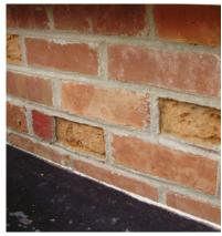
[2] **Not Recommended:** The use of inappropriate Portland cement mortar to repoint these soft 19th-century bricks has caused some of them to spall. *Photo: Courtesy Nebraska State Historic Preservation Office.*
