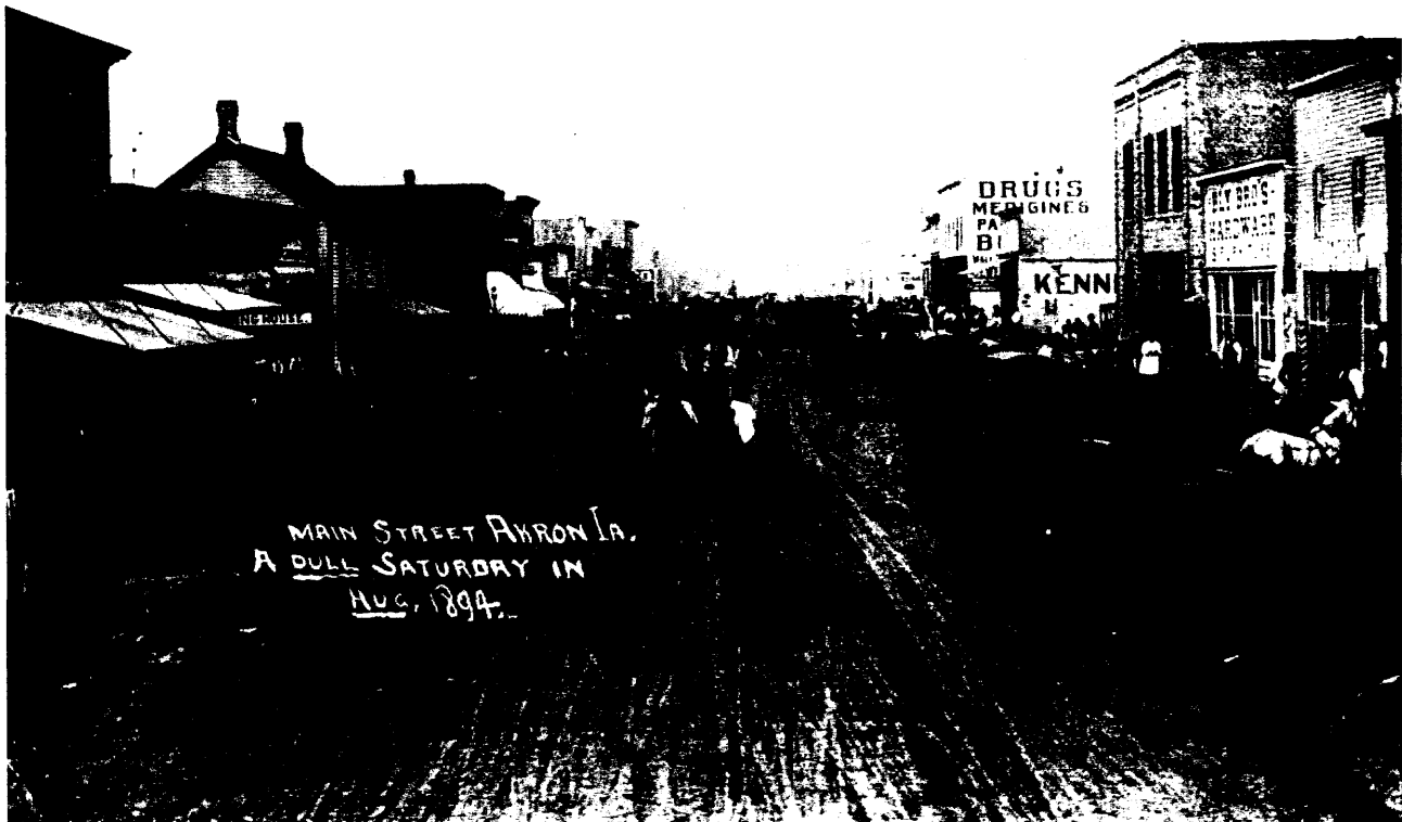
“A Dull Saturday ” in Akron, Iowa, on the border with South Dakota, 1894. Though most buildings are still wooden false-fronts, a few substantial masonry buildings have been constructed. The large building on the right, next to “Bly Bro’s Hardware” has a façade of stone ashlar that changes to brick for the sidewall construction. From SHSI, IC; reprinted in Bennett, 280.
