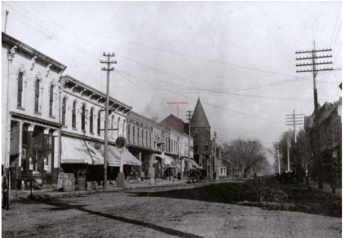
Image 01. Historic Image - View looking north along S. Dubuque Street - 1893
