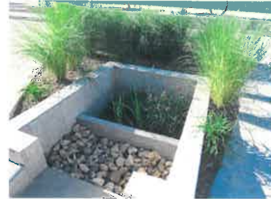
Improvements to 5th Street in Coralville included green infrastructure to filter stormwater.
