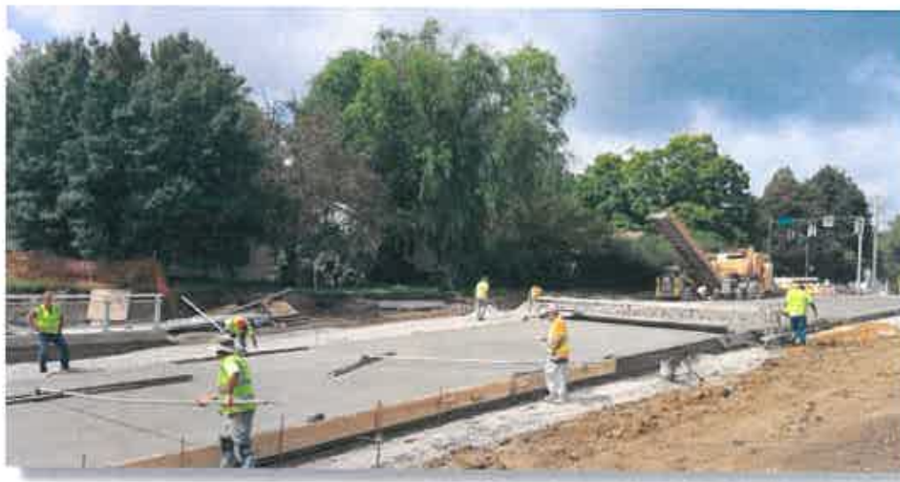
Reconstruction of First Avenue for grade separation under the Iowa Interstate Railroad.
